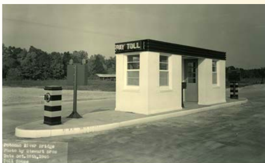
1940 Maryland toll plaza
