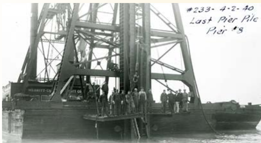
Last pile driven, 1940
