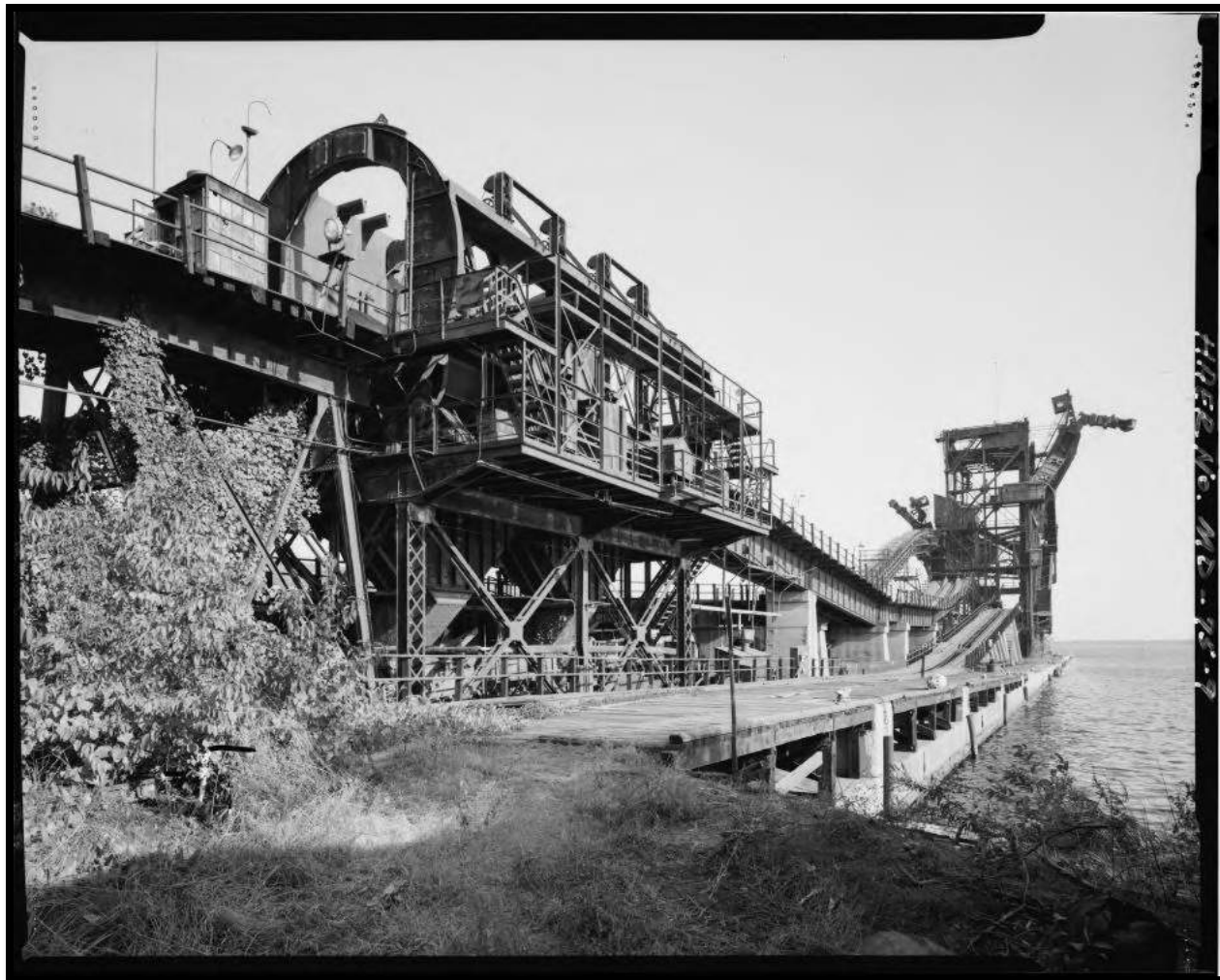
Port Covington coal pier. Credit: Library of Congress, Prints & Photographs Division, HAER, HAER MD,4-BALT,190--9
