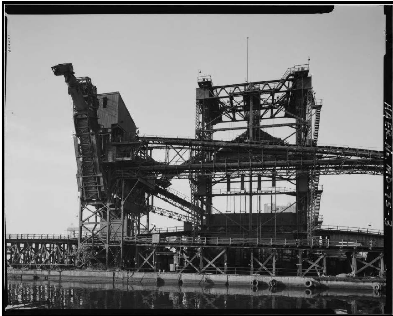
Port Covington coal pier. Credit: Library of Congress, Prints & Photographs Division, HAER, HAER MD,4-BALT,190—3
