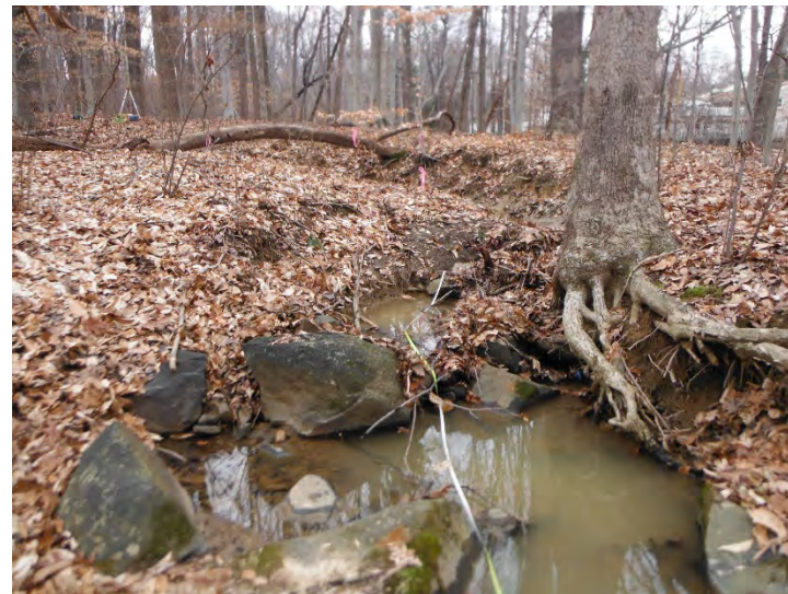
Close-up view upstream at boulder knick point (~Sta. 6+90).
