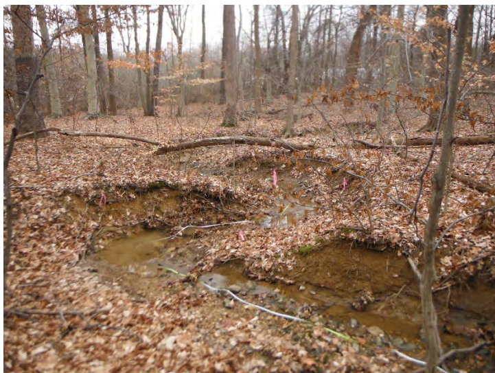
Facing downstream from Sta. 6+20 at typical Reach 3 bank erosion and point bars.
