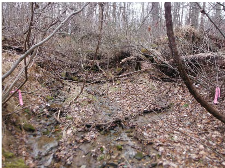
Facing upstream at debris jam / knick point (break between Reach 1&2)
