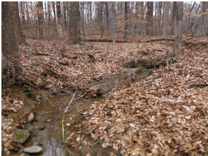
Facing upstream from station 7+75. Photo shows alternating point bars, right bank erosion, and boulder knick point.
