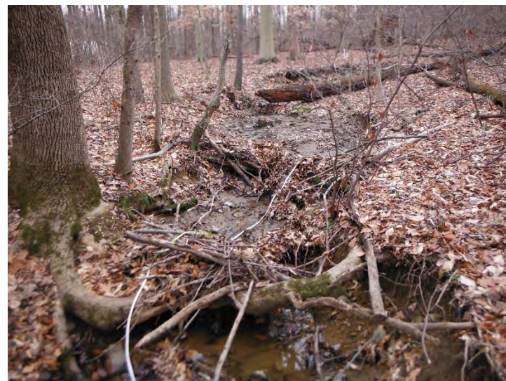
Facing upstream at 2 foot knick point between Reaches 2 & 3.
