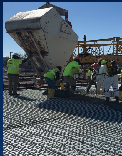
Crews working on pre-cast decks.
