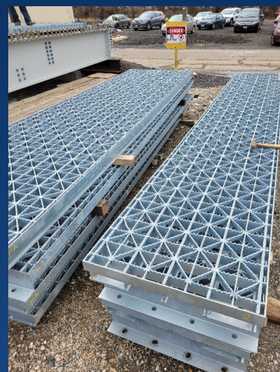
Temporary joint grates.
