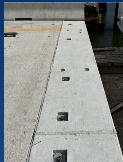
Temporary concrete connection slabs.
