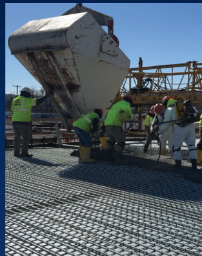
Crews working on pre-cast decks.
