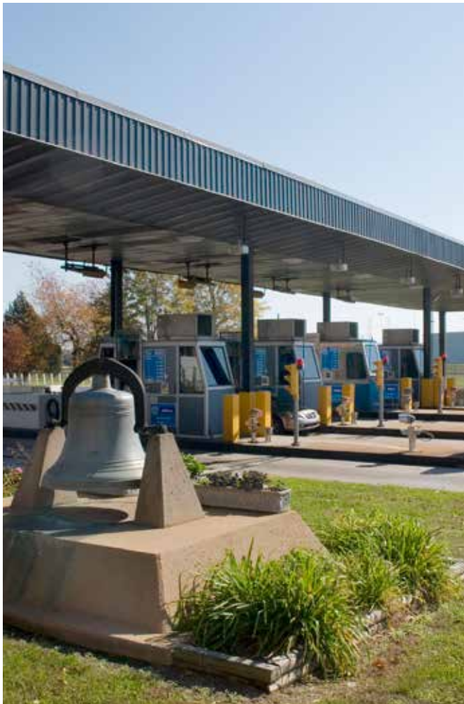
Nice Bridge Toll Plaza
