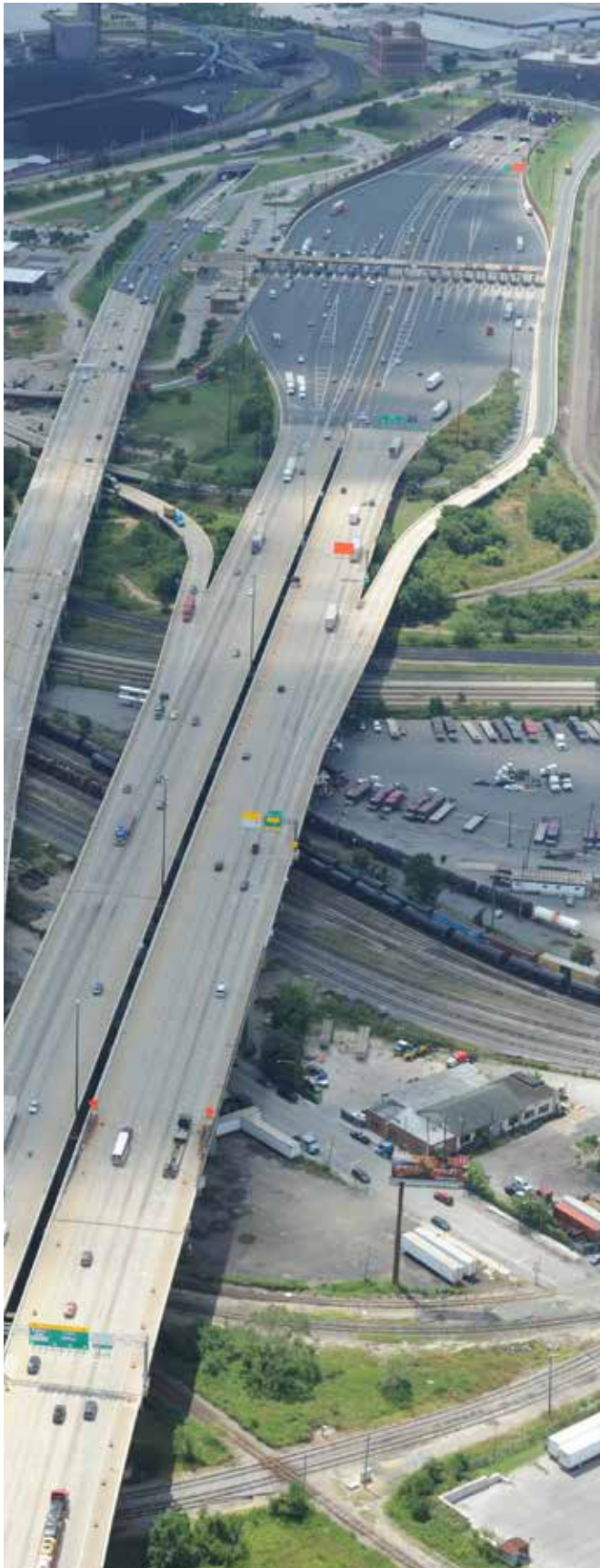
Fort McHenry Tunnel approach roadway and toll plaza
