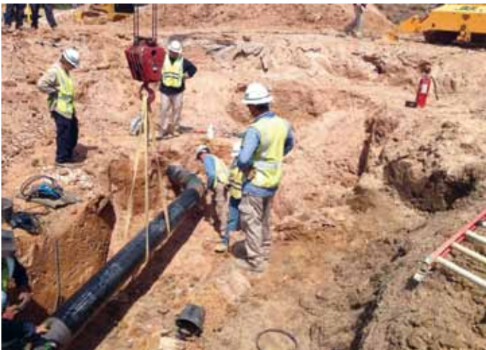
I-95 Express Toll Lanes at MD 43 Interchange, BGE Gas Line Relocation
