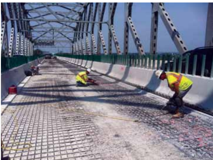
I-895 K-Truss Bridge Redecking
