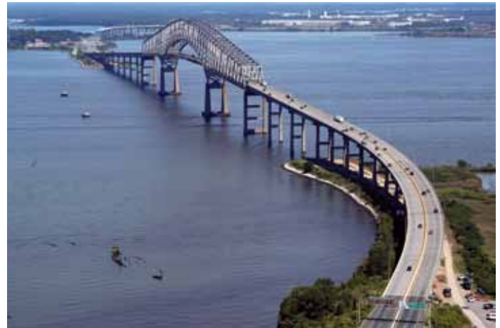
Francis Scott Key Bridge (I-695)
