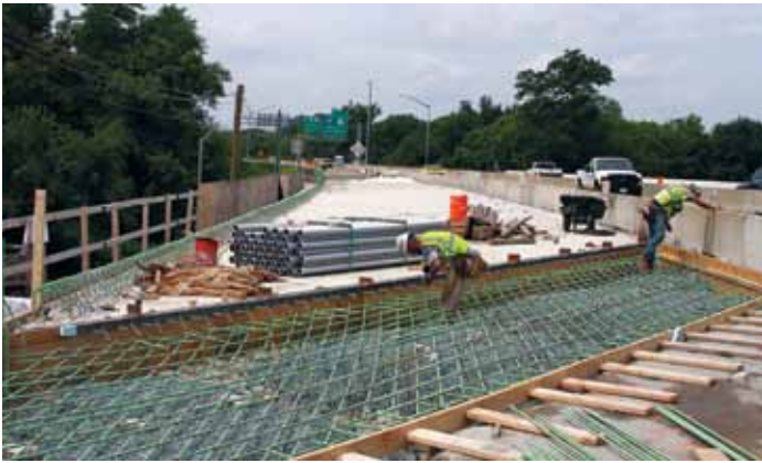
Patapsco Avenue Bridge Decking
