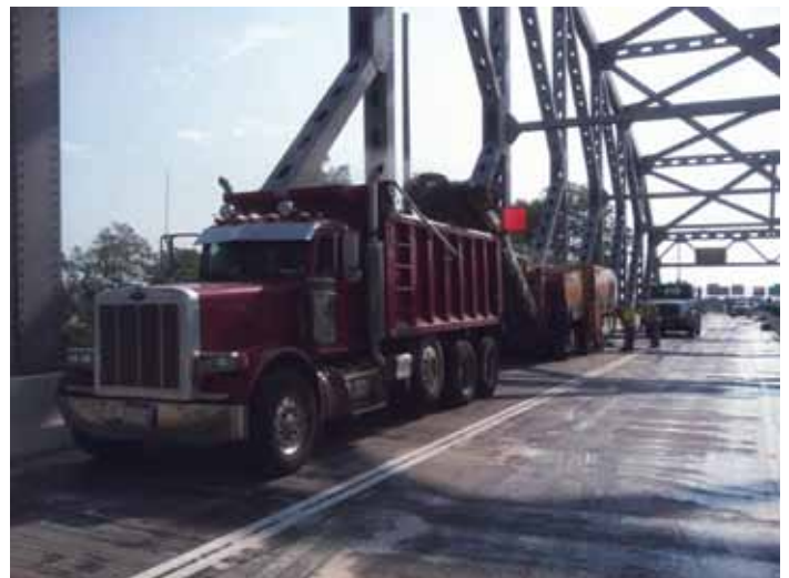
I-895 K-Truss Bridge Redecking
