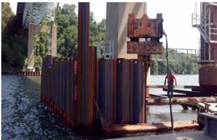
I-95 Tydings Bridge Pier Cofferdam
