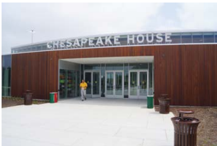
I-95 CHESAPEAKE HOUSE TRAVEL PLAZA
