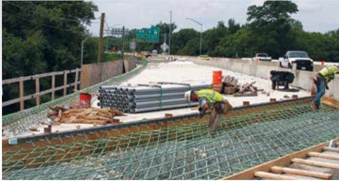
PATAPSCO AVENUE BRIDGE RE-DECKING PROJECT ON I-895 (BALTIMORE HARBOR TUNNEL)
