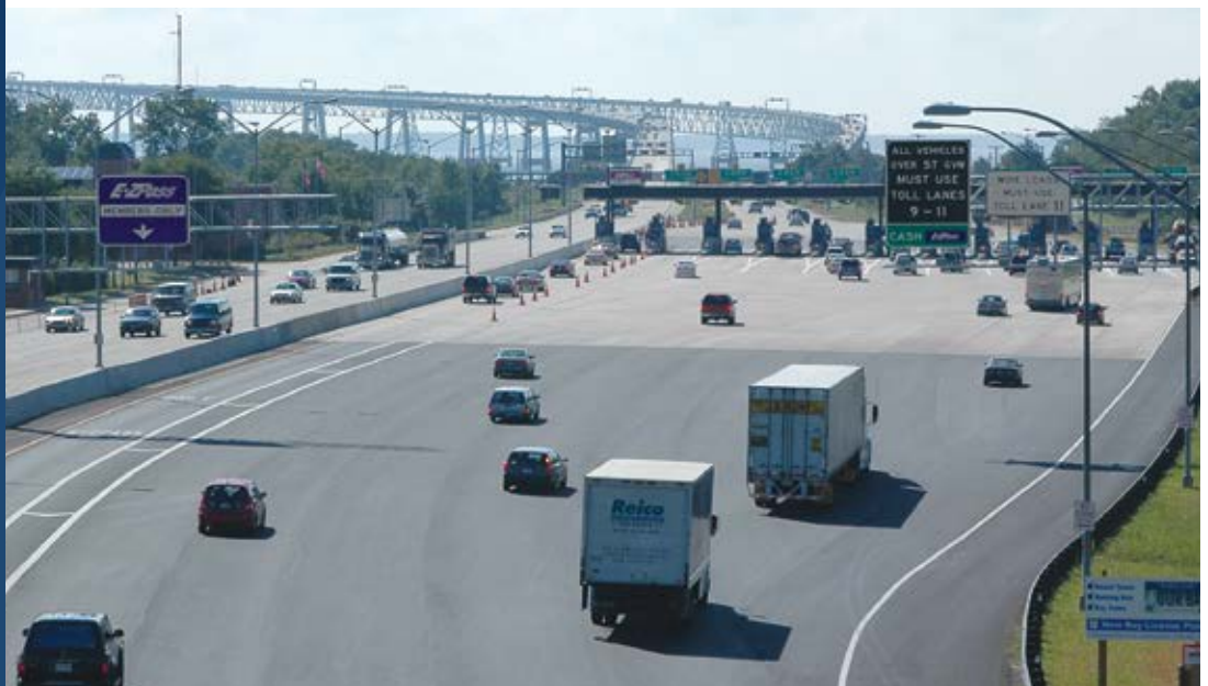
WILLIAM PRESTON LANE JR., MEMORIAL (BAY) BRIDGE (US 50/301)
