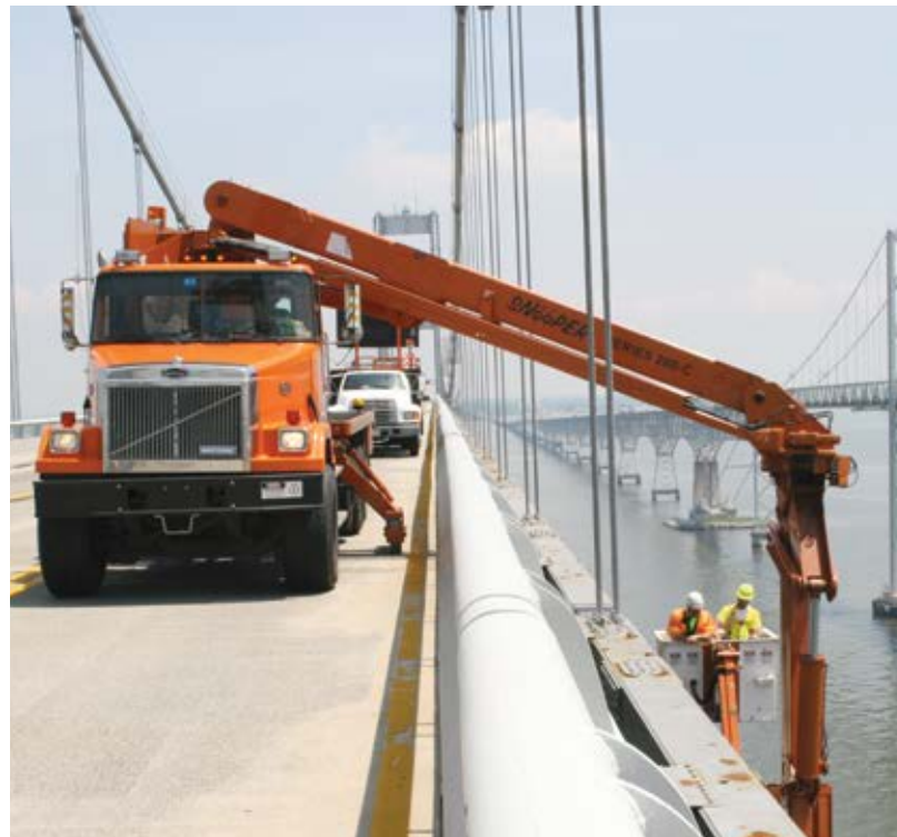
BAY BRIDGE FACILITY INSPECTION
