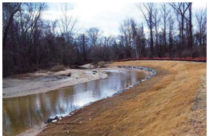
STREAM BANK STABILIZATION AREA AFTER CONSTRUCTION
