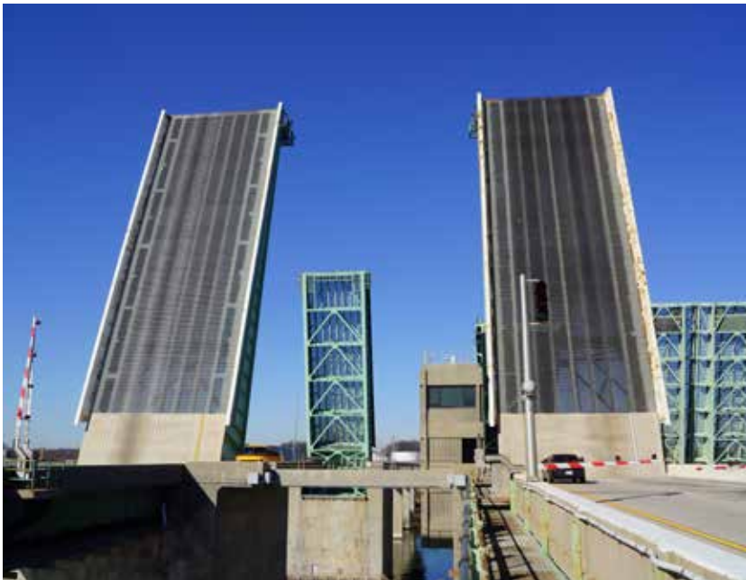
CURTIS CREEK DRAWBRIDGE
