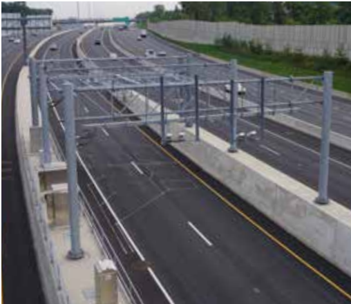
ABOVE: I-95 EXPRESS TOLL LANES
