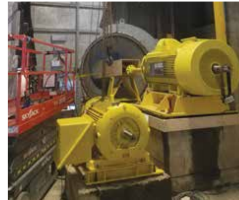
ABOVE: NEW VENTILATION FANS BEING INSTALLED AT THE HARBOR TUNNEL LEFT: BAY BRIDGE PAINTING
