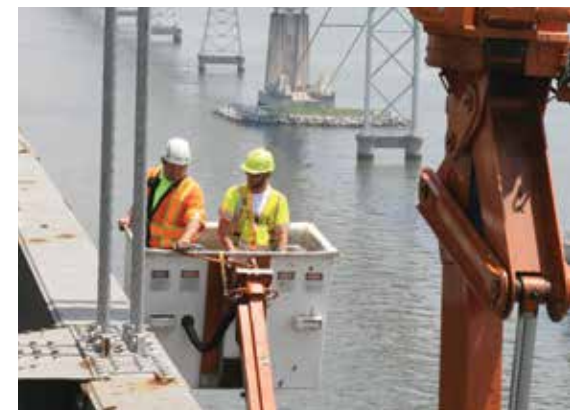
BELOW: BAY BRIDGE SUSPENSION SPAN REHABILITATION
