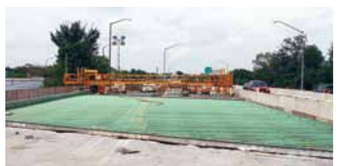
► Hanover Street bridge decking
