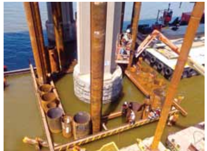
► Thomas J. Hatem Memorial Bridge foundation and substructure
