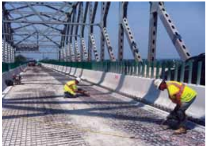
► K-Truss Bridge at the Baltimore Harbor Tunnel (I-895)
