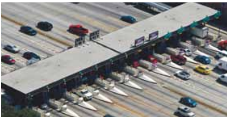
► Baltimore Harbor Tunnel toll plaza
