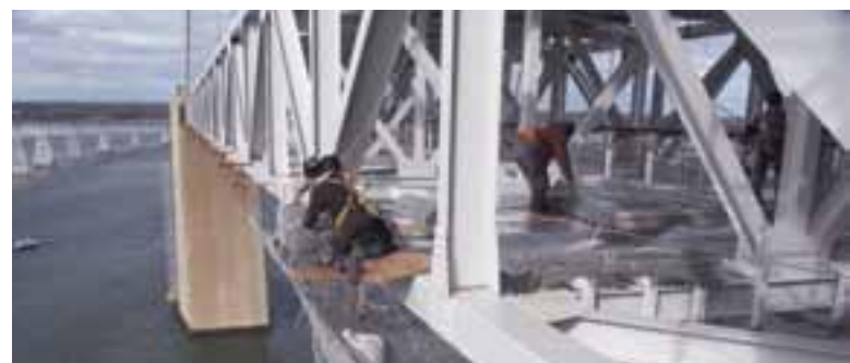
▶ Crews assemble the containment system for the Bay Bridge painting project.
