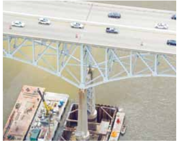
► Millard E. Tydings Memorial Bridge substructure
