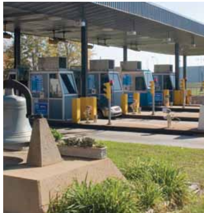
▶ Gov. Harry W. Nice Memorial (Potomac River) Bridge toll plaza
