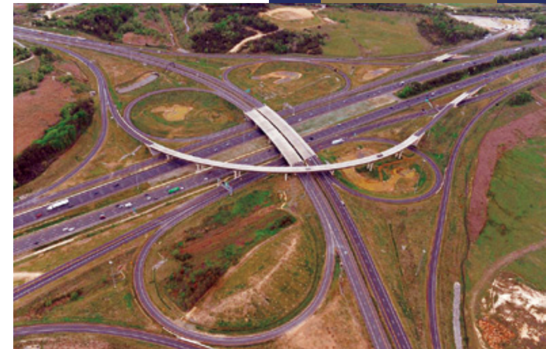
The ICC interchange at Interstate 95 in Prince George's County.
