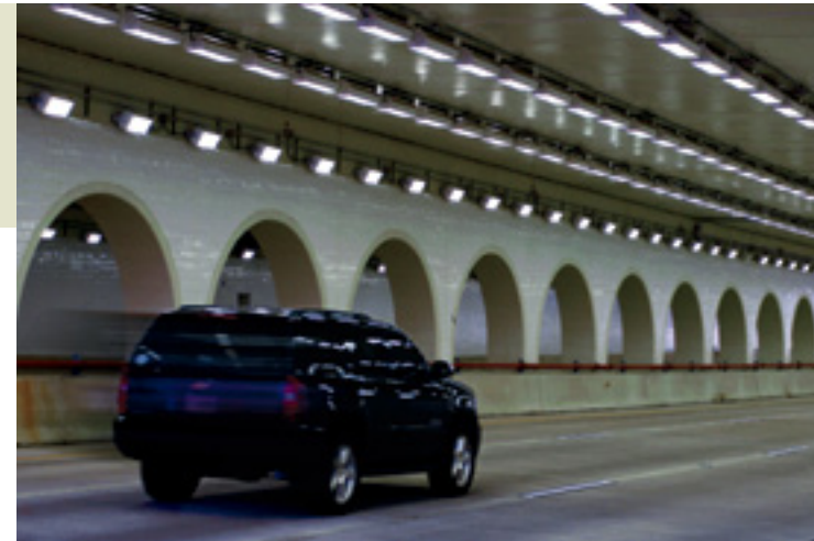
ICC traffic travels below Olde Mill Run.
