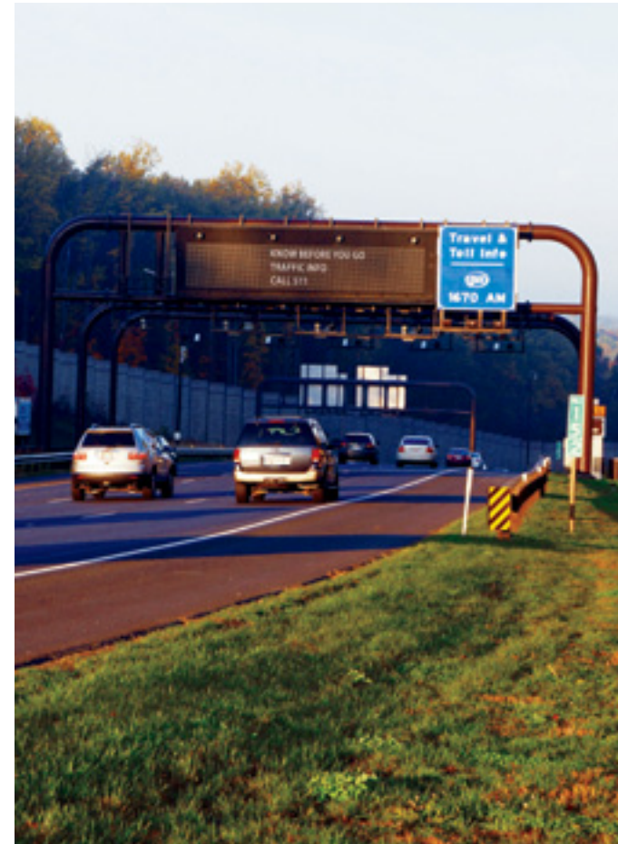
Overhead tolling gantry along the Intercounty Connector (ICC)/MD 200.
