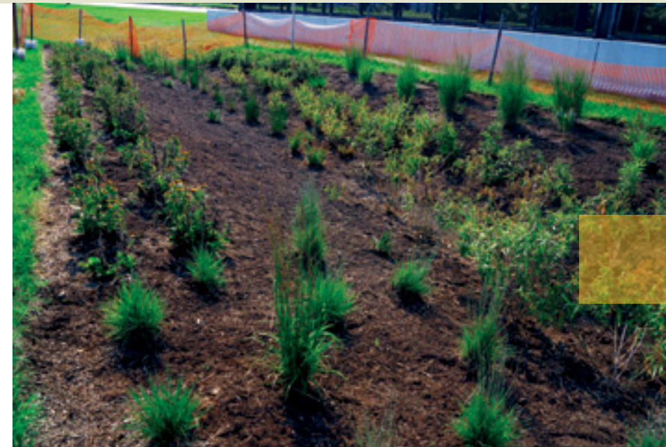
The Fort McHenry Tunnel Rain Garden.
