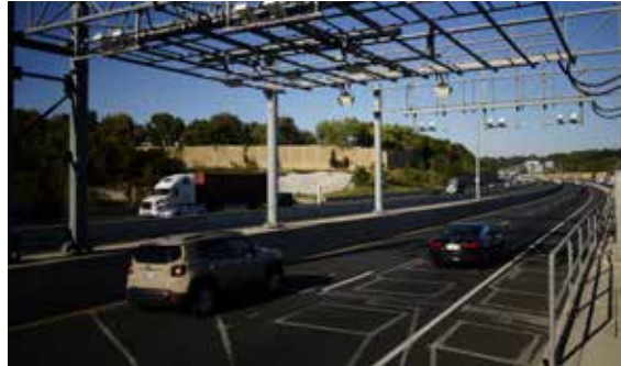
I-95 EXPRESS TOLL LANES
