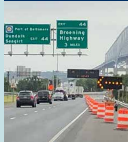
MAINTENANCE OF TRAFFIC DEVICES AT THE KEY BRIDGE
