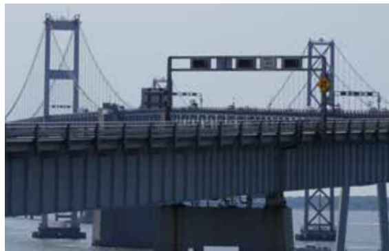
WESTBOUND BAY BRIDGE REHABILITATION
