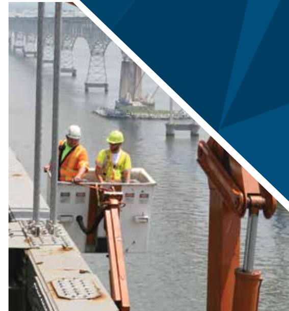
Bay Bridge Painting
