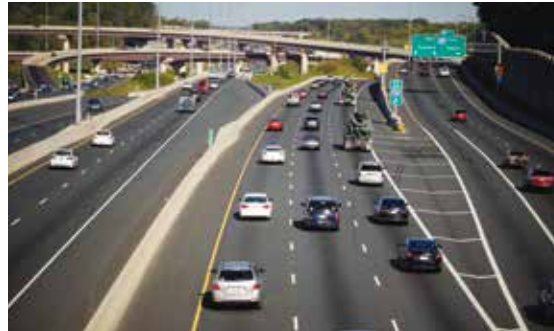
I-95 Express Toll Lanes
