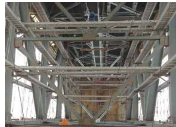
Bay Bridge Suspension Span Rehabilitation
