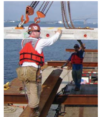
New through truss deck sections en route to the Bay Bridge.
