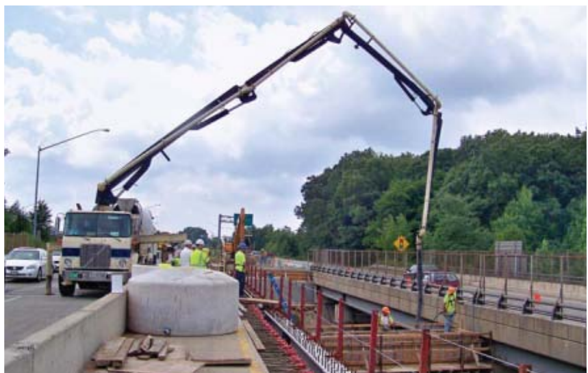
Widening of MD 24 bridge over I-95.
