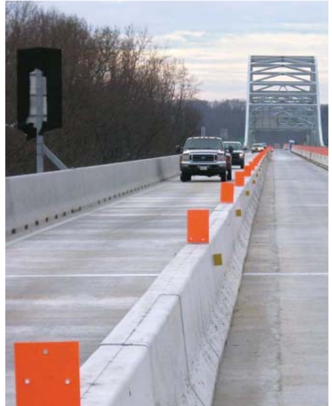
Completed eastbound redecking.
