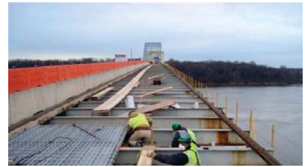
Setting grid for eastbound redecking.
