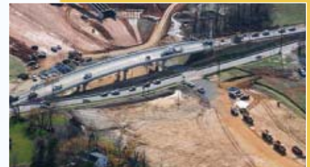
The new Old Columbia Pike bridge.
