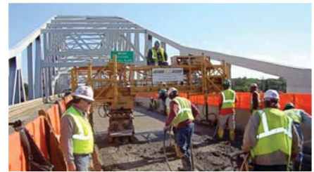
Pouring concrete onto new grid.
