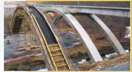
Signature Arch Bridge over Rock Creek.
