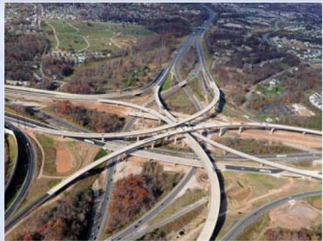
Aerial view of new I-95/I-695 interchange ramps.
