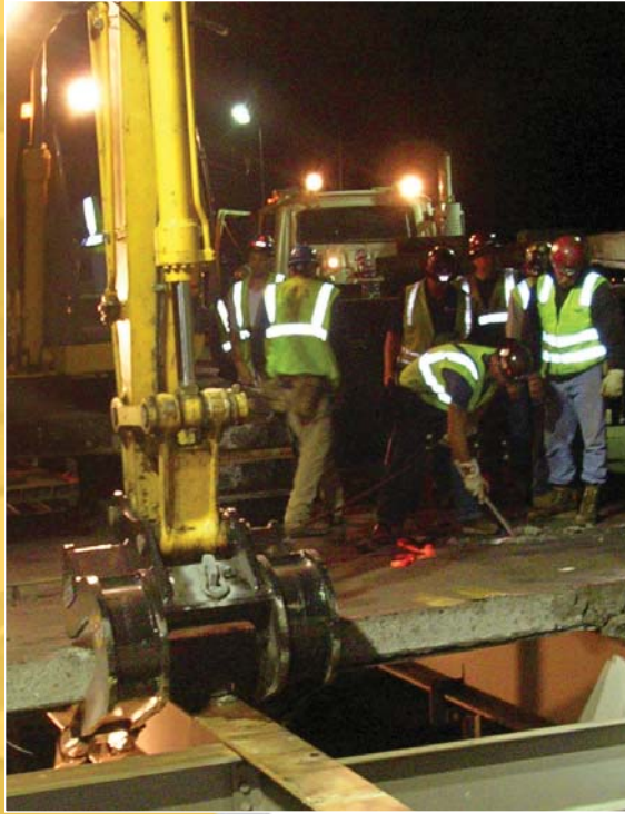
Through truss deck removal with concrete crab.
