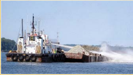
Concrete from Bay Bridge redecking created the reef foundation.
