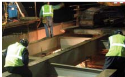
Crews clean steel stringers before new deck is installed.
