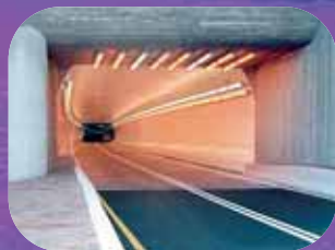
Fort McHenry Tunnel (I-95, I-395)
