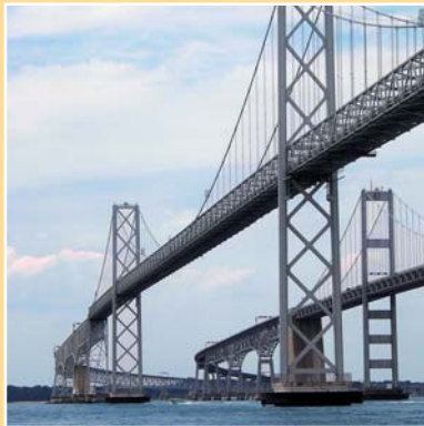
William Preston Lane Jr. Memorial (Bay) Bridge (US 50/301)
