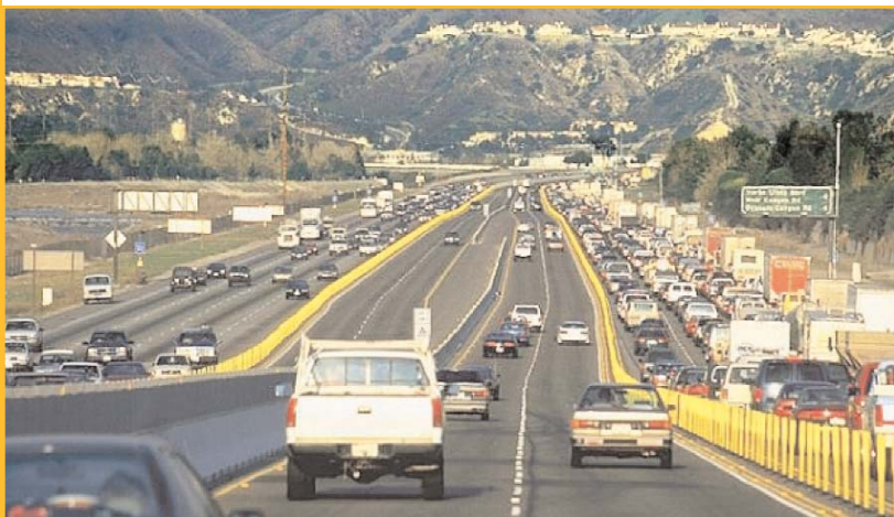
SR 91, Orange County, Calif. Toll Managed Lanes (Center), Free Lanes (Right) (Note: All ICC lanes to be managed using tolls - no free lanes)
