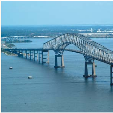
Francis Scott Key Bridge (I-695)
