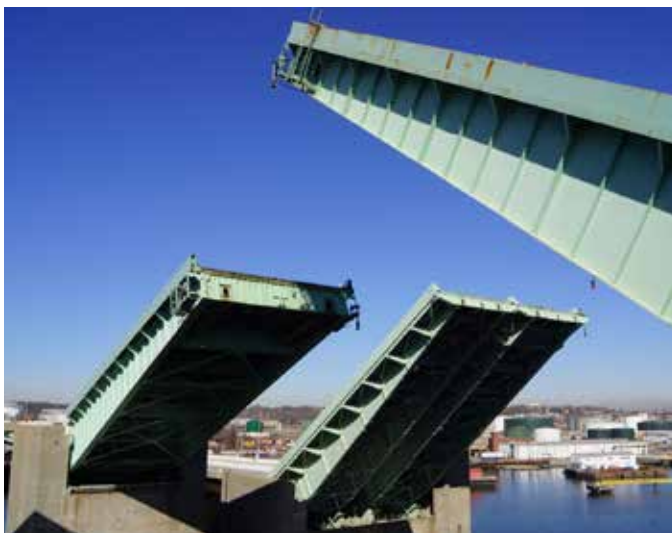
Curtis Creek Drawbridge (I-695)
