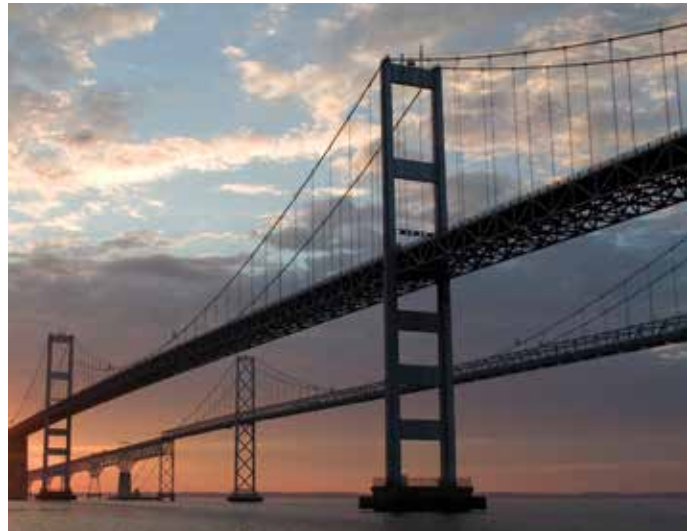
William Preston Lane, Jr. Memorial (Bay) Bridge (US 50/301)
