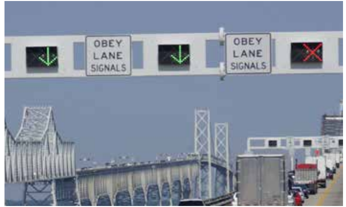
Overhead Lane Use Signals at the Bay Bridge
