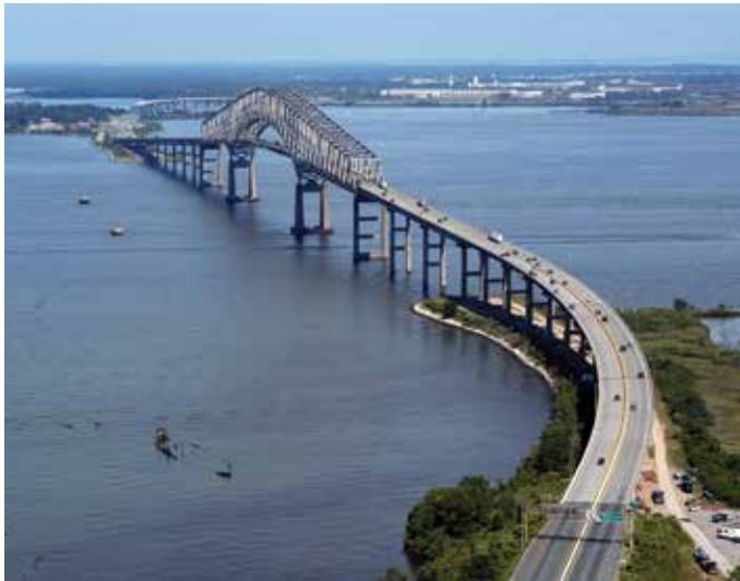
Francis Scott Key Bridge (I-695)
