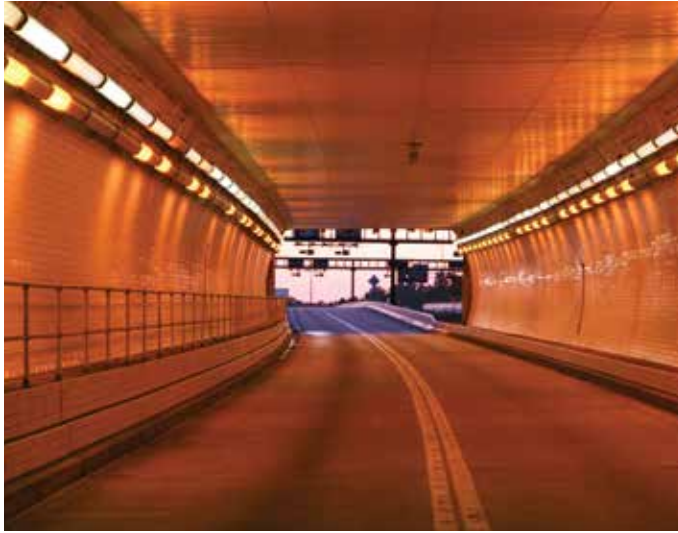
Fort McHenry Tunnel (I-95, I-395)
