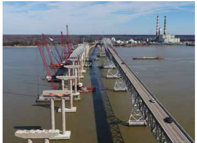
Building the new Nice/Middleton Bridge.
