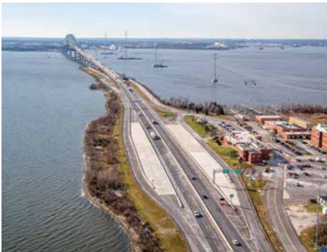
Aerial view of the Key Bridge Facility.
