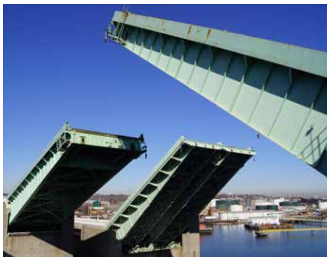
Curtis Creek Drawbridge (I-695)
