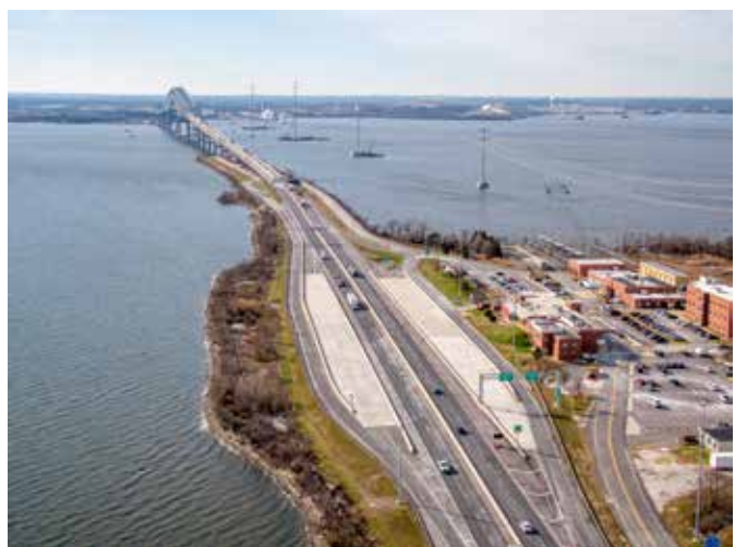
Aerial view of Key Bridge Facility
